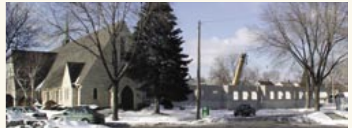
The new $4.5 million Garden Homes Lutheran School under construction.
